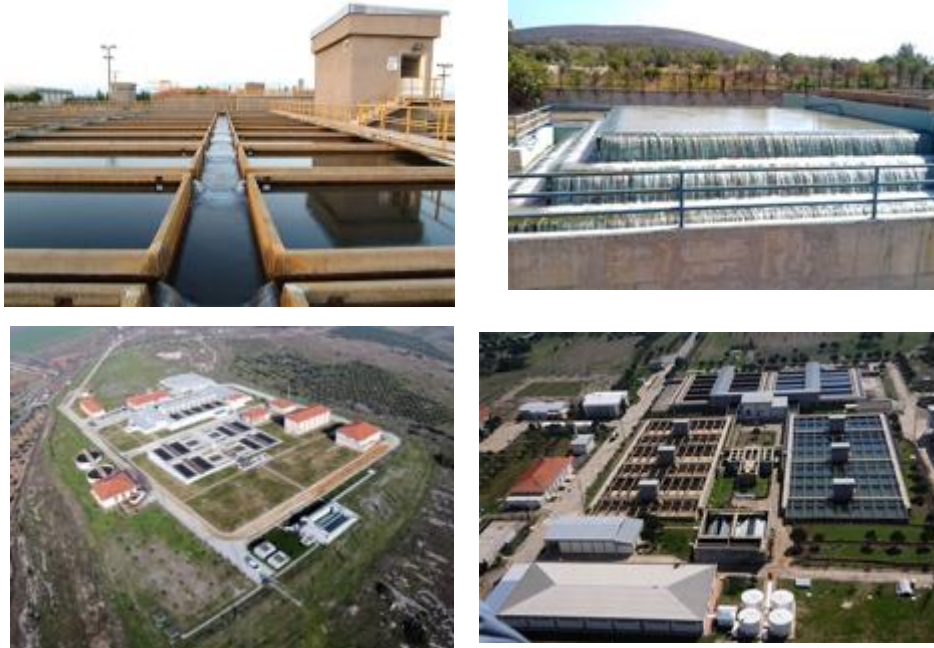
Views from potable water treatment plants in İzmir
