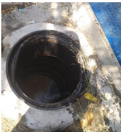
Closed grit chamber system for pre-treatment of wastewater to be discharged to the sewer system (Central Campus)
