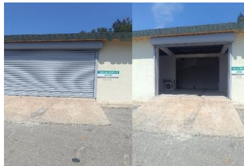
Hazardous waste temporary storage areas at DEU campuses
