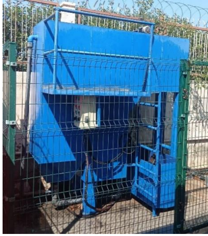
Closed grit chamber systems for pre-treatment of wastewater to be discharged to the sewer system (15 Temmuz Health and Art Campus)
