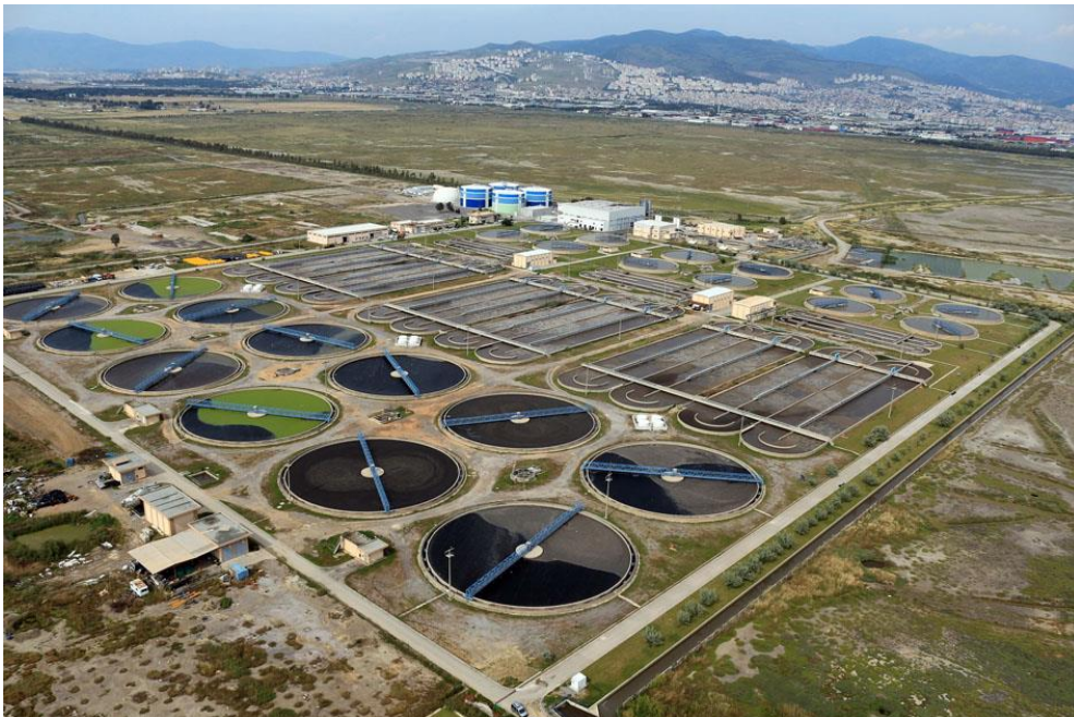
IZSU Wastewater Treatment Plant for Izmir city
