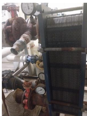
Geothermal Exchangers in 15 Temmuz Health and Art Campus
