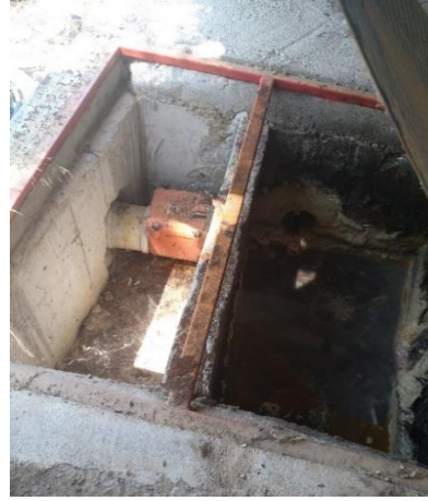
Closed grit chamber systems for pre-treatment of wastewater to be discharged to the sewer system (15 Temmuz Health and Art Campus)
