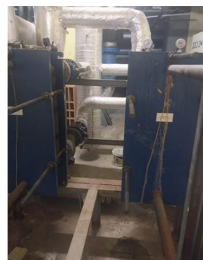
Geothermal Exchangers in 15 Temmuz Health and Art Campus
