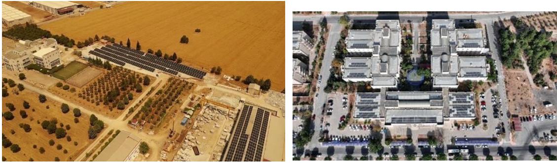
Solar energy pannels from DEU
