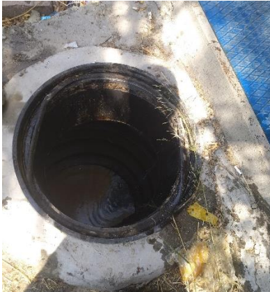
Closed grit chamber system for pre-treatment of wastewater to be discharged to the sewer system (Tınaztepe Central Campus)
