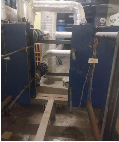
Geothermal Exchangers in 15 Temmuz Health and Art Campus
