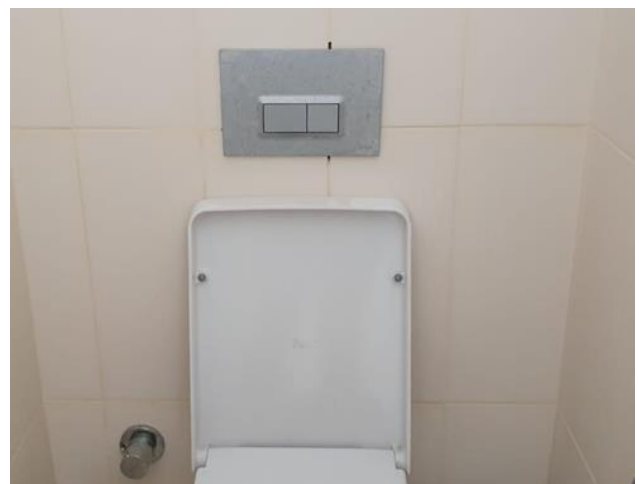
Double stage system reservoirs
