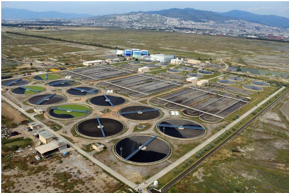
IZSU Wastewater Treatment Plant for Izmir city
