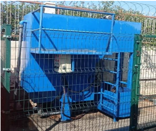
Closed grit chamber systems for pre-treatment of wastewater to be discharged to the sewer system (15 Temmuz Health and Art Campus)
