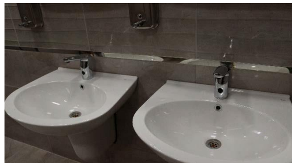
Use of photocell taps in various DEU Campuses
