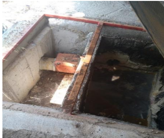
Closed grit chamber systems for pre-treatment of wastewater to be discharged to the sewer system (15 Temmuz Health and Art Campus)
