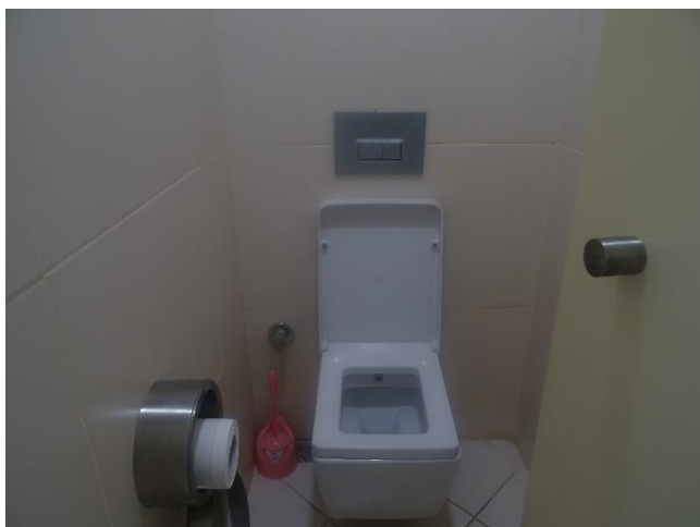
Double stage system reservoirs
