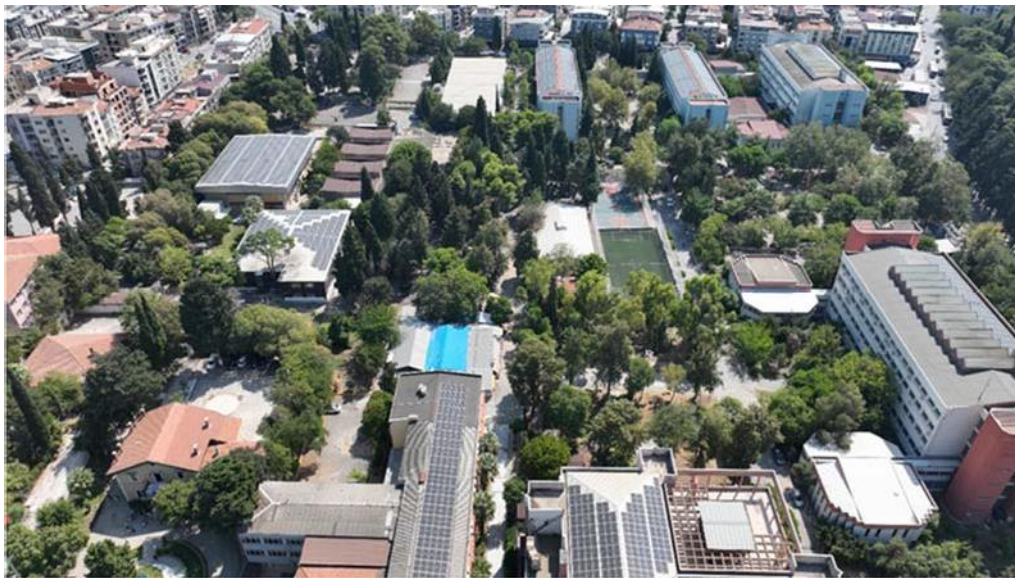
Solar energy pannels in Dokuzçesmeler Campus of DEU
