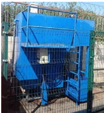
Closed grit chamber systems for pre-treatment of wastewater to be discharged to the sewer system (15 Temmuz Health and Art Campus)
