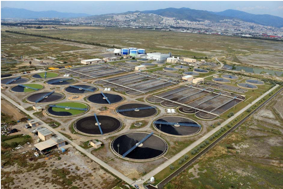
IZSU Wastewater Treatment Plant for Izmir city
