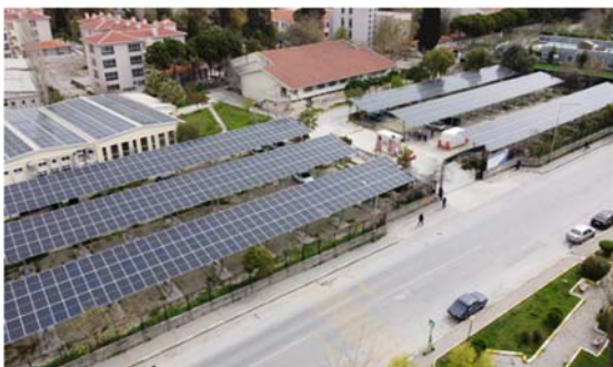
Solar energy pannels from Education Faculty
