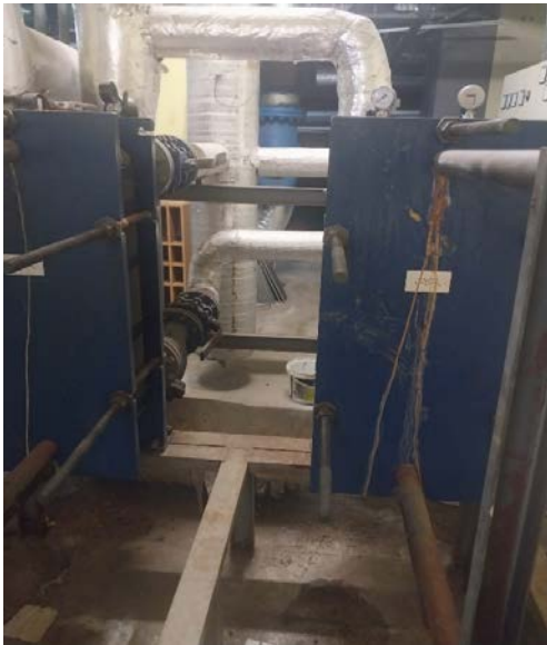
Geothermal Exchangers in 15 Temmuz Health and Art Campus
