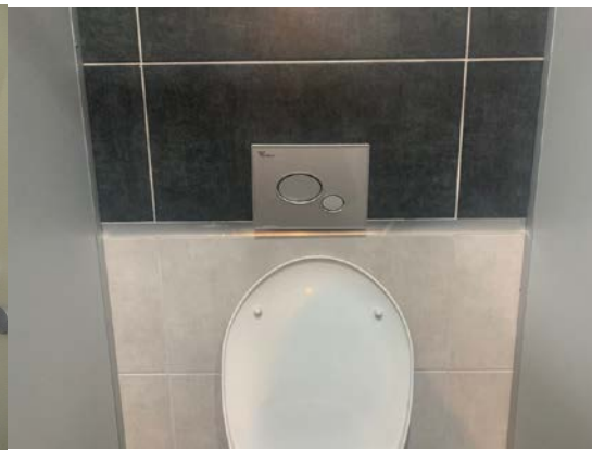
Use of double-stage reservoir systems in various DEU Campuses
