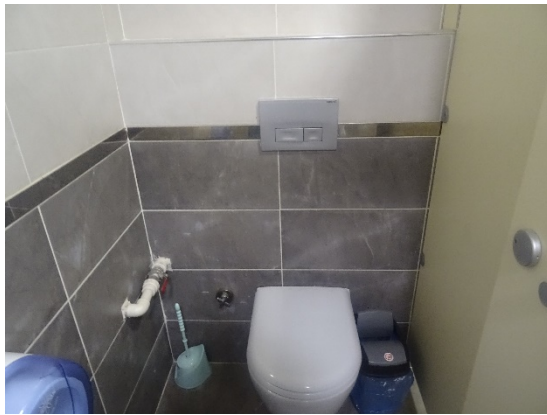
Use of double-stage reservoir systems in various DEU Campuses
